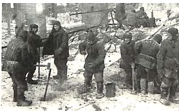
Prisoners building a copper factory in Norilsk in 1949
